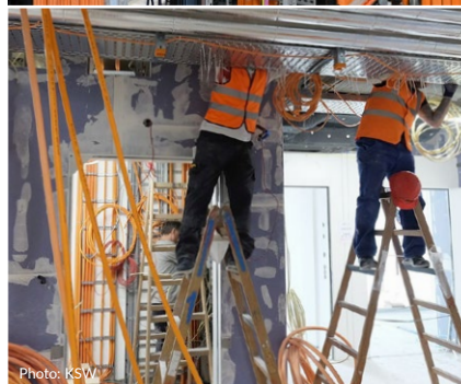
Around 1,000 km of electric cables were laid for the new building.
