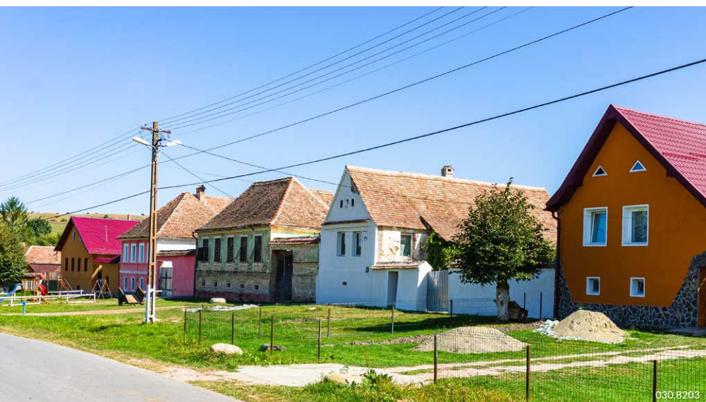
Increasingly better fiber optic supply in rural areas thanks to aerial deployment
